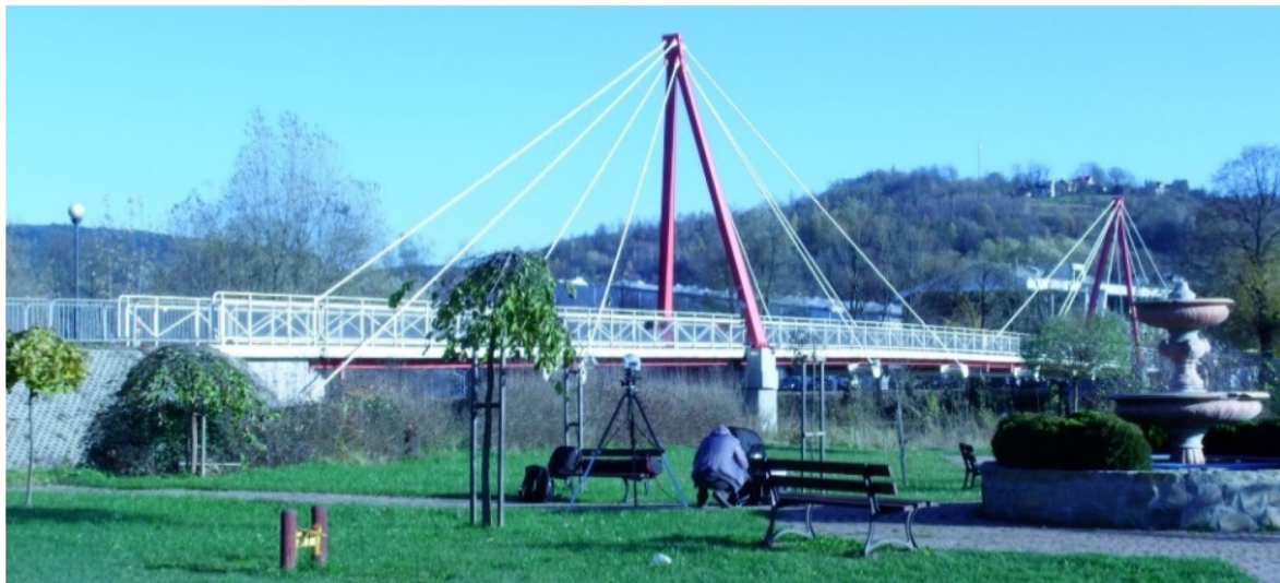
Fig. 5 In-field experimental tests of the footbridge: (a) configurations of measurement points; (b) RSV-150 laser Doppler vibrometer
